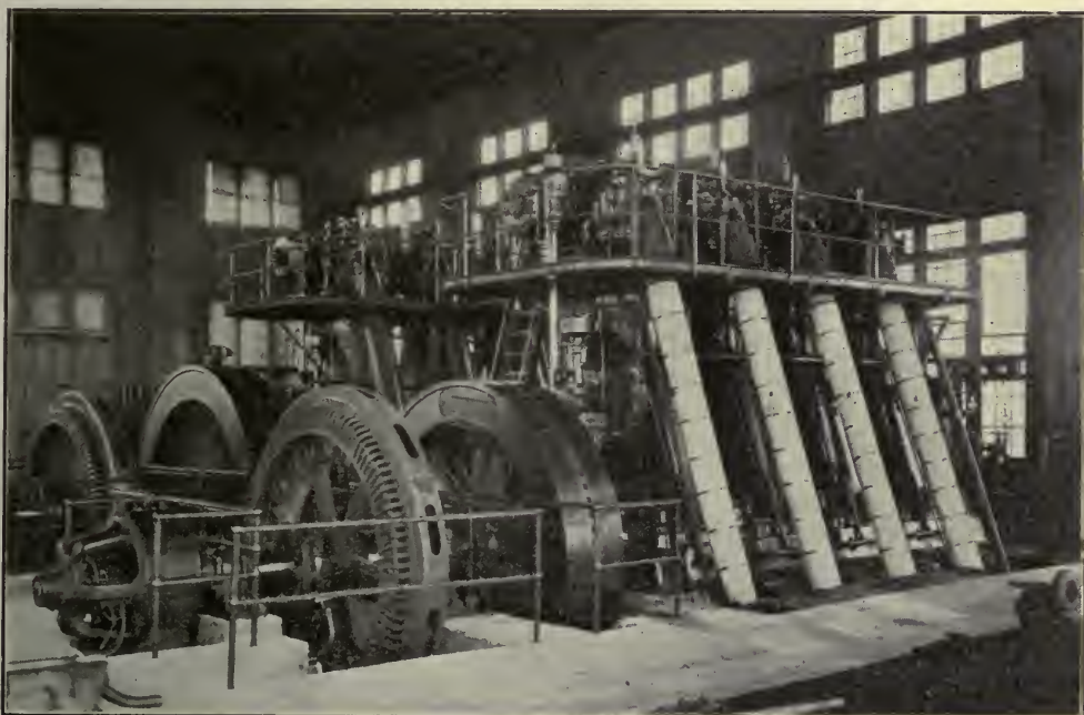
INTERIOR VIEW OF POWER-PLANT, SHOWING INSTALLATION OF DIESEL ENGINES
